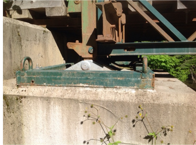
left bank bearing
