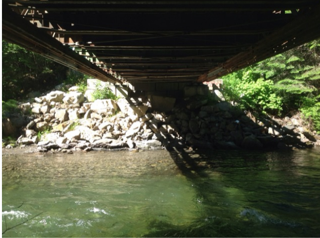
Left Bank Abutment when facing downstream
