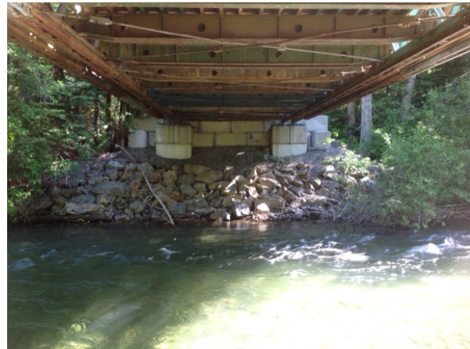
Right Bank Abutment when facing downstream
